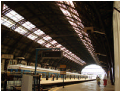
Fig 8 Retiro Railway Station – Buenos Aires 1915
